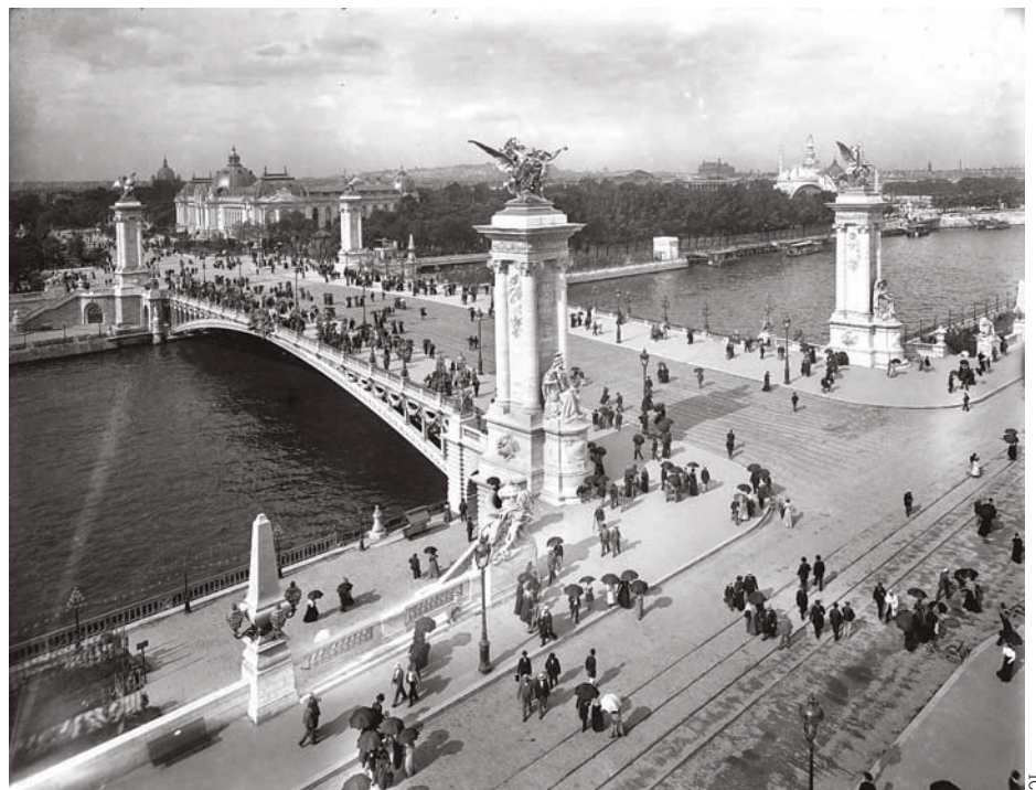
Paris' elaborate Pont Alexandre III, built in preparation for the 1900 Universal Exposition
