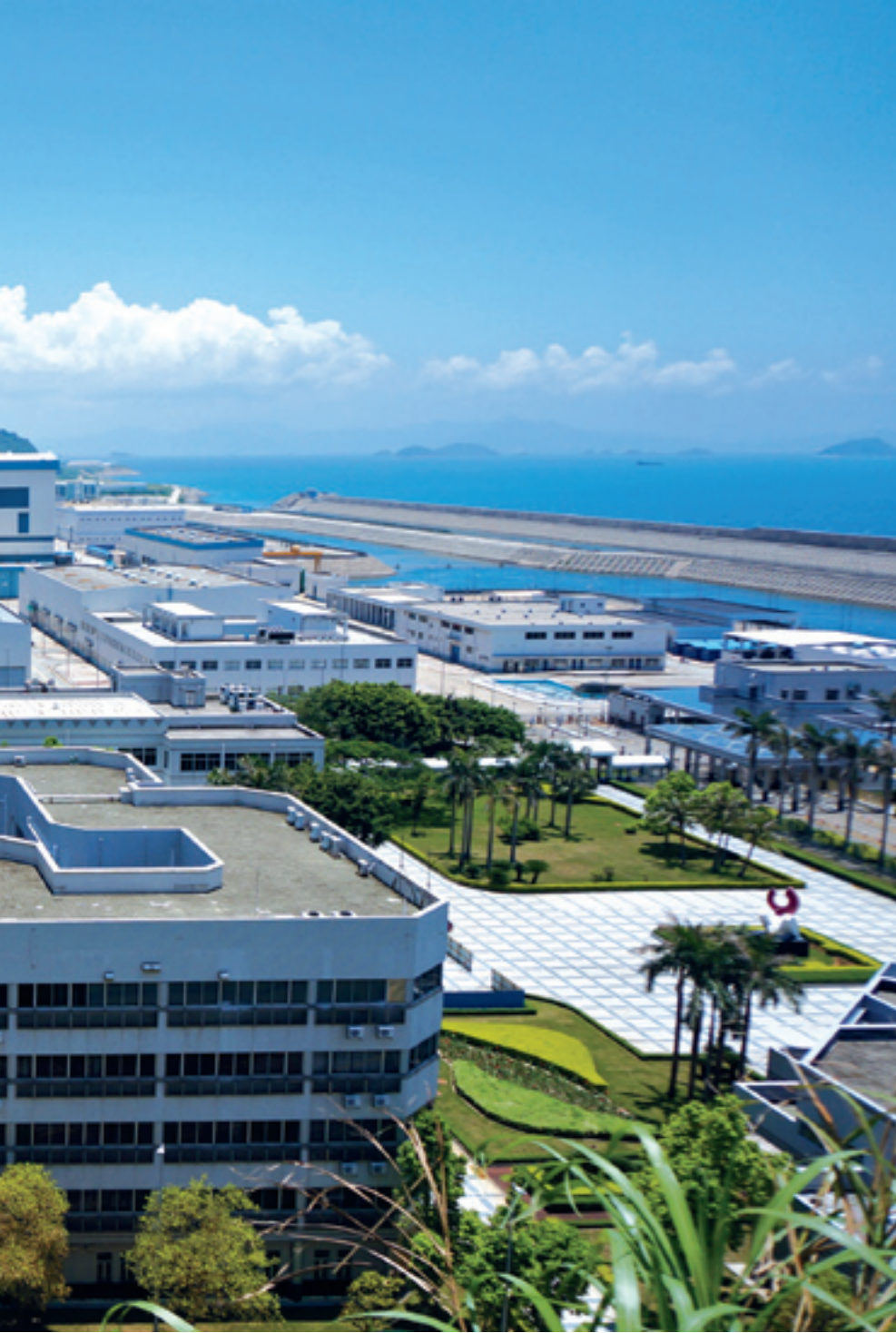
CLEAN ELECTRICITY: Pictured is Phase 1 of the Ling'ao power plant, which has two nuclear reactors that came into commercial operation respectively in 2002 and 2003
