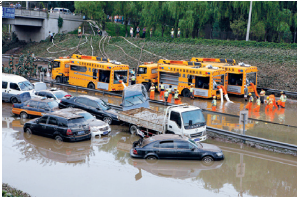
LONG RESCUE EXPRESS: Workers and soldiers pump water out of a submerged section of the Beijing-Hong Kong-Macao Expressway the day after the flood on July 22
