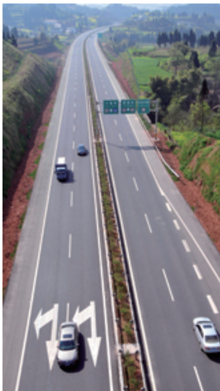
NEW CONNECTION The expressway linking Guangyuan and Nanchong of southwest China's Sichuan Province opens on April 1. The 201-km expressway halves the travel time between the two cities to two hours
