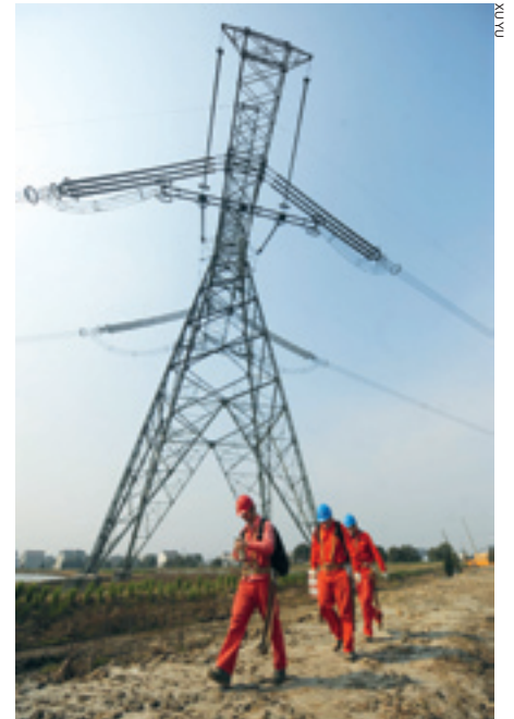
POWERLINE PATROL Workers inspect \pm 800 KV Ultra High Voltage transmission lines in Huzhou, east China's Zhejiang Province, on March 13. The transmission project traverses eight provinces with a total length of 2,089 km
