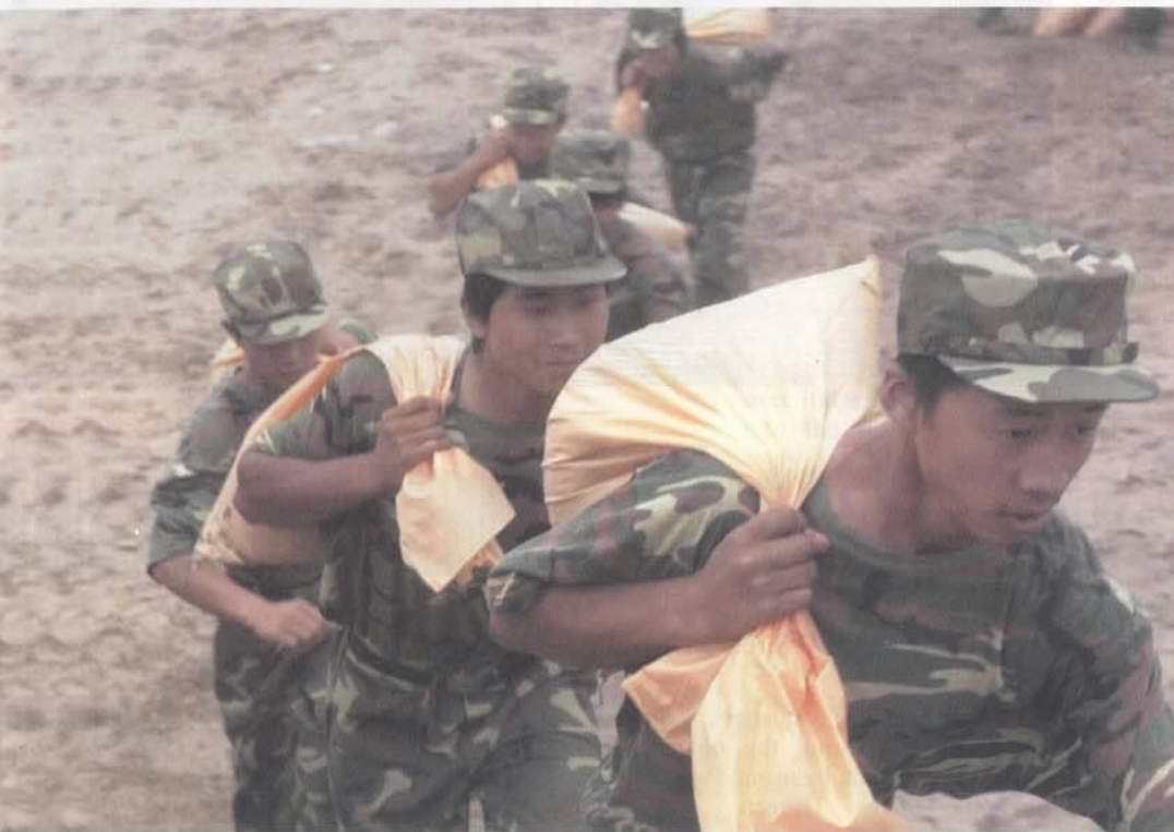
STEMMING THE TIDE: Soldiers carry the load as they rush with sandbags to reinforce a flooded dyke
